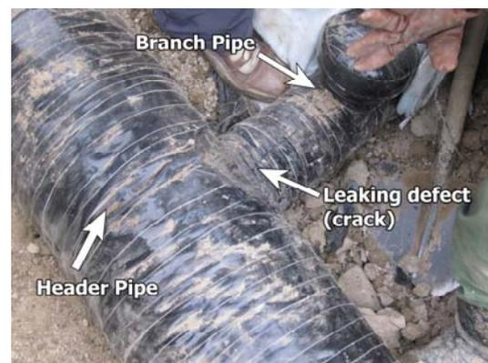
**Figure 1.** Split sleeve for branch connection repairs
